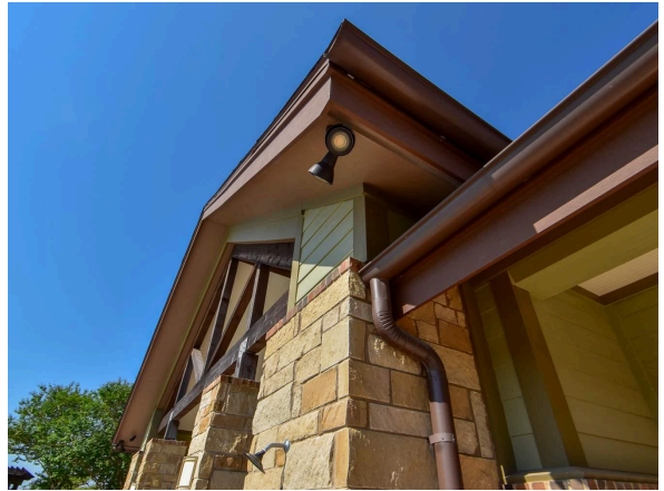
Pool house exterior surfaces and rain gutters
