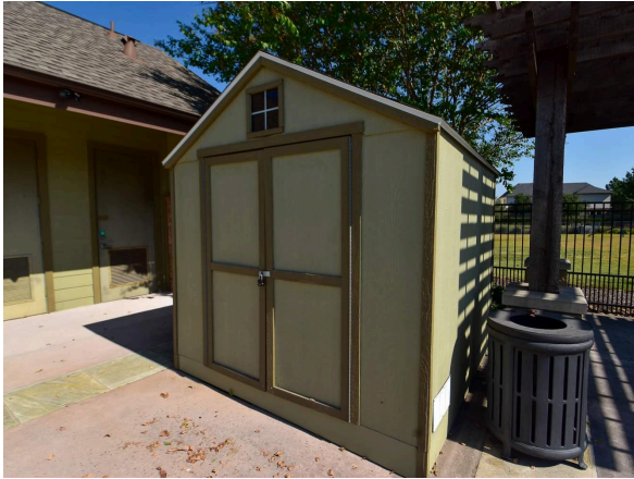
Pool area shed
