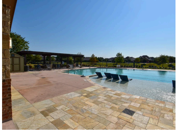
Pool concrete and pavers deck
